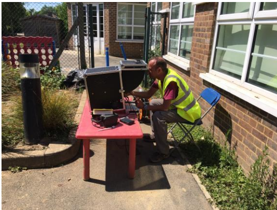
Figure 2. HD CCTV camera void surveys set up
